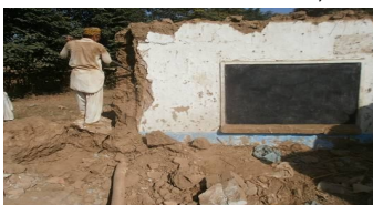
Demolishing of classroom in progress at BEFARe School (MSB 008)
