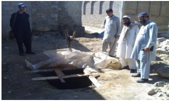
Likore well bore at site-2 completed
