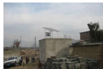
Mandezo well bore at site-1 completed
