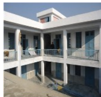
A view of newly constructed class room of GPS
