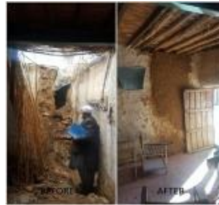
A view of classroom before and after repair work
