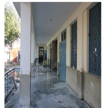
Outer Structure of Newly constructed class rooms under RAHA project
